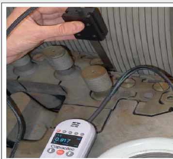
PowerGen - rotor to stator
